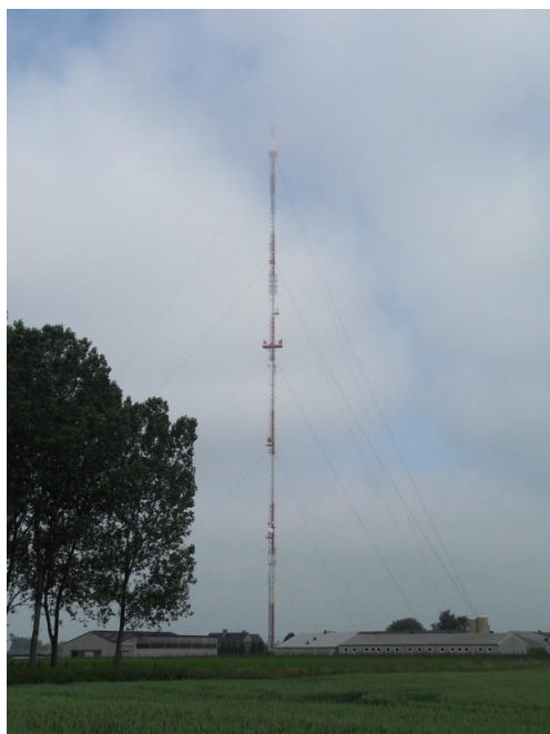
De VRT-mast in Egem
