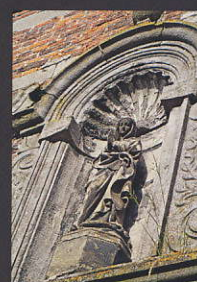
Detail of the Façade
